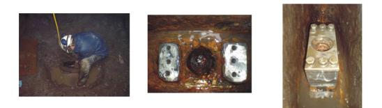
Figure 2: Valve gate prepared for attachment of new spindle nut carrier blocks
