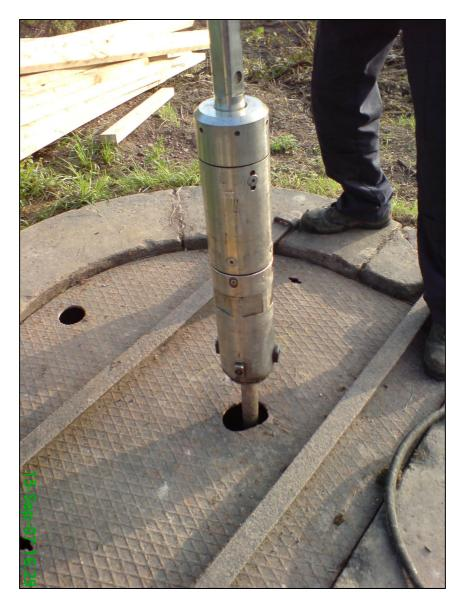
Figure 3: Typical H-Grip set up to release a seized valve
